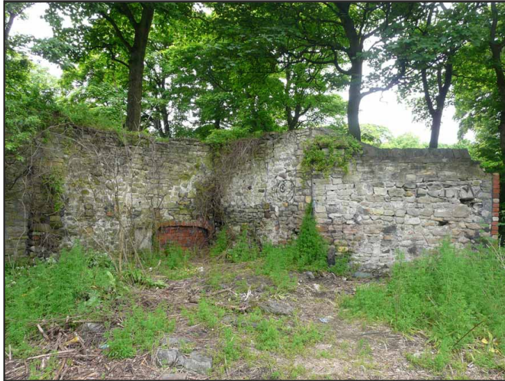
Illus. 28: Blocked door at the east end of the north wall of the former tithe barn.
