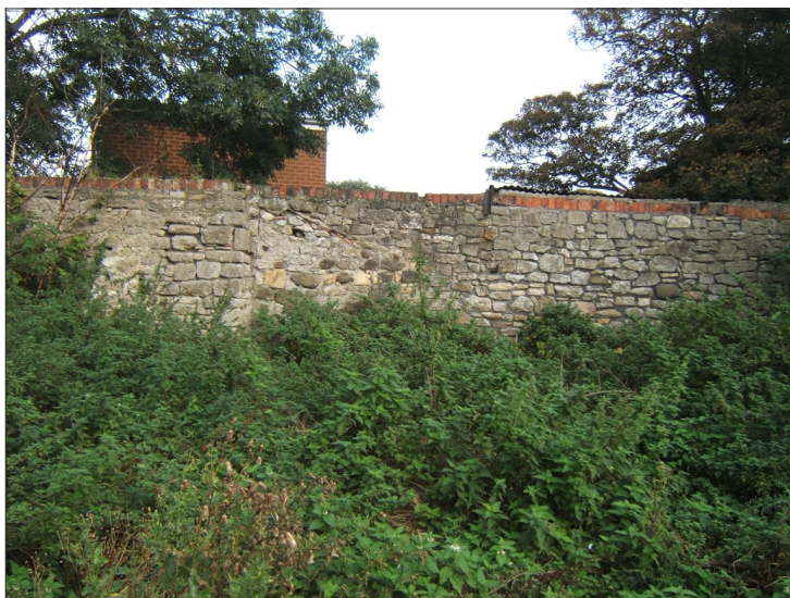
Illus, 27: Part of the east wall of the assessment site (note former roof line in central section).
