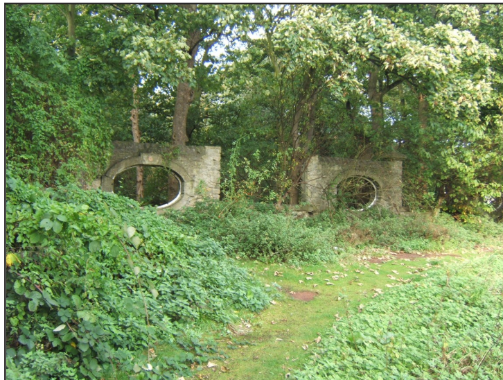
Illus. 29: West part of the east-west wall within the assessment site - showing oval openings constructed around 1900 (photographed prior to the collapse of the near-side opening).
